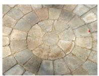
Manufactured Pavers come in many sizes, including a special mix that creates a radius pattern like this one.
