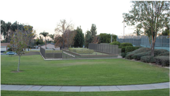
City of Corona Department of Water and Power Manglar Blending Facility HDR
