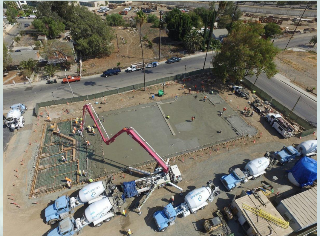
PLACING BUILDING FLOOR CONCRETE
