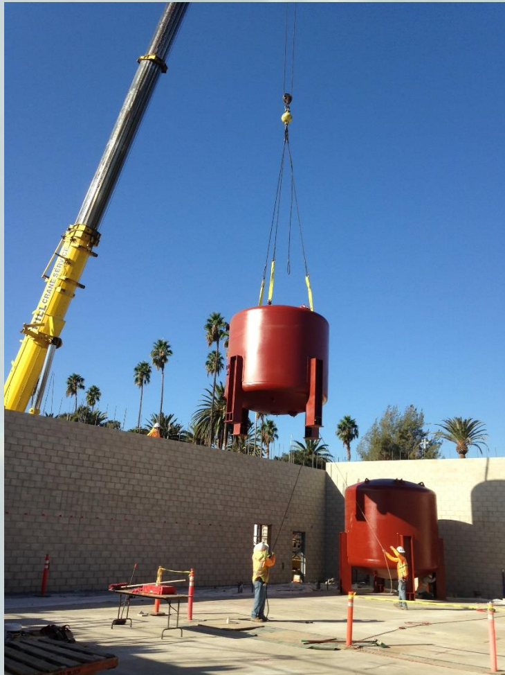
DELIVERY OF TREATMENT VESSEL
