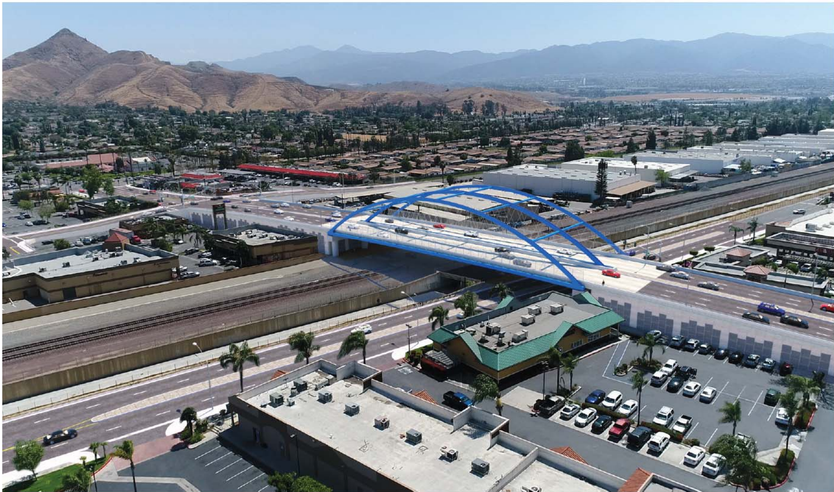
MCKINLEY STREET OVERPASS
