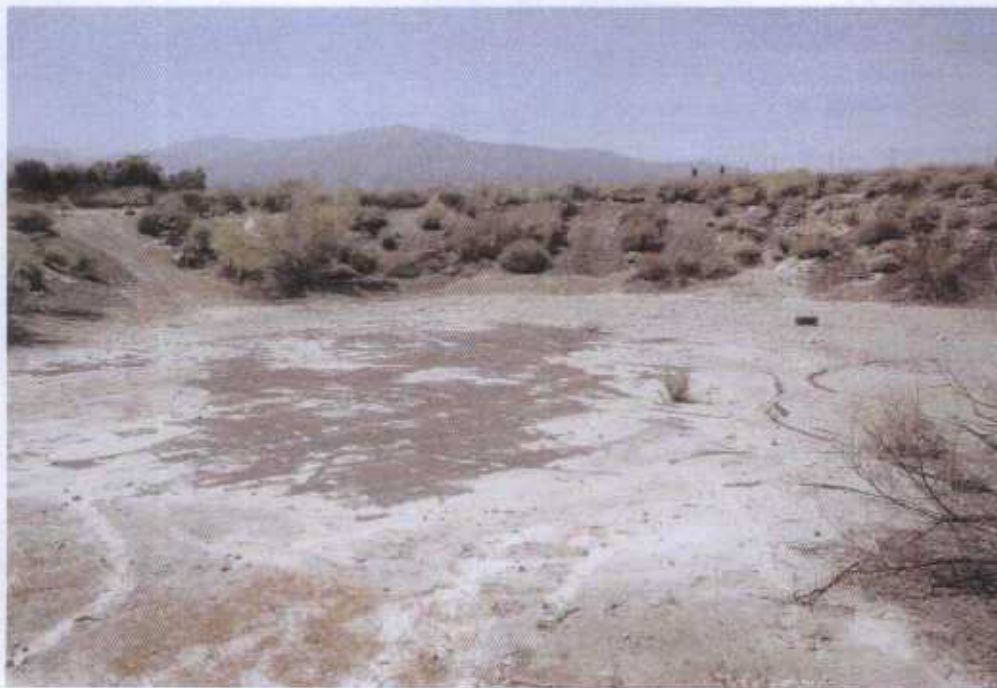
PHOTOGRAPH 6 - View facing north of non-jurisdictional isolated remnant agricultural pond. When the pond was constructed, it was lined with asphalt or tar which is still present, along with sediment that has entered the depressional area from adjacent upper areas. Riversidean sage scrub surrounds the edge.
