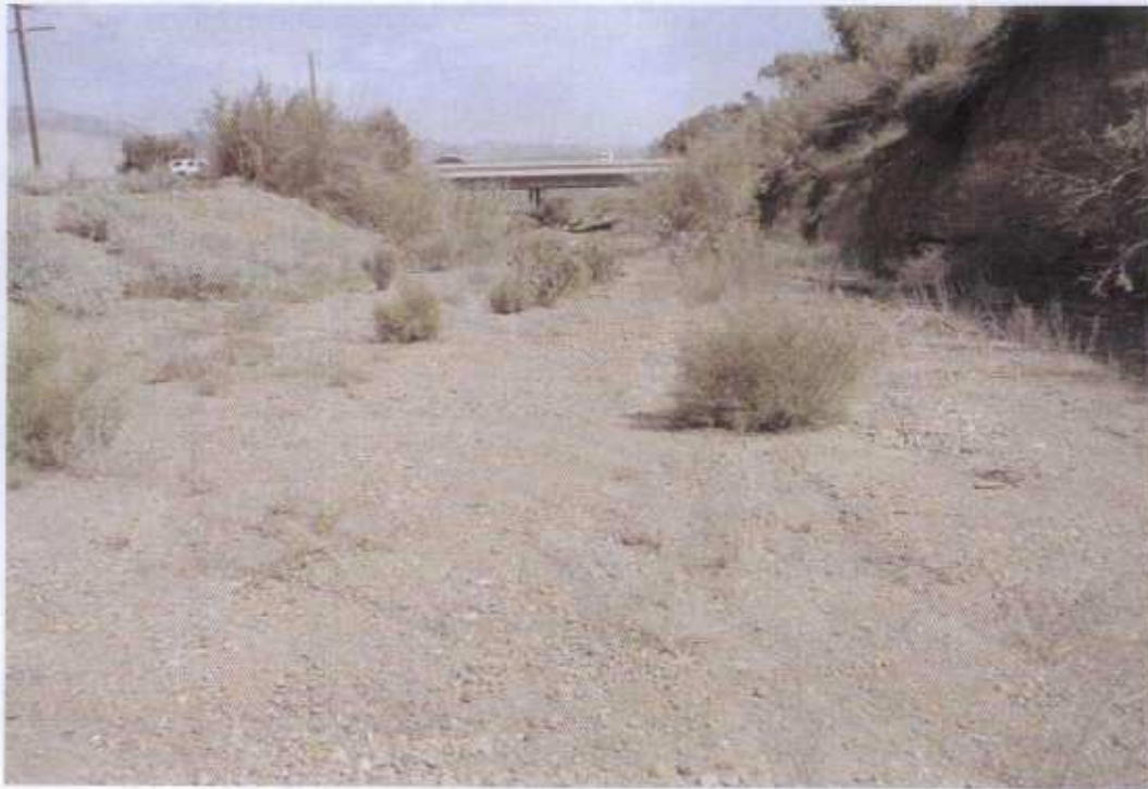
Photograph 4 depicts the predominantly unvegetated streambed within Bedford Canyon Wash.
