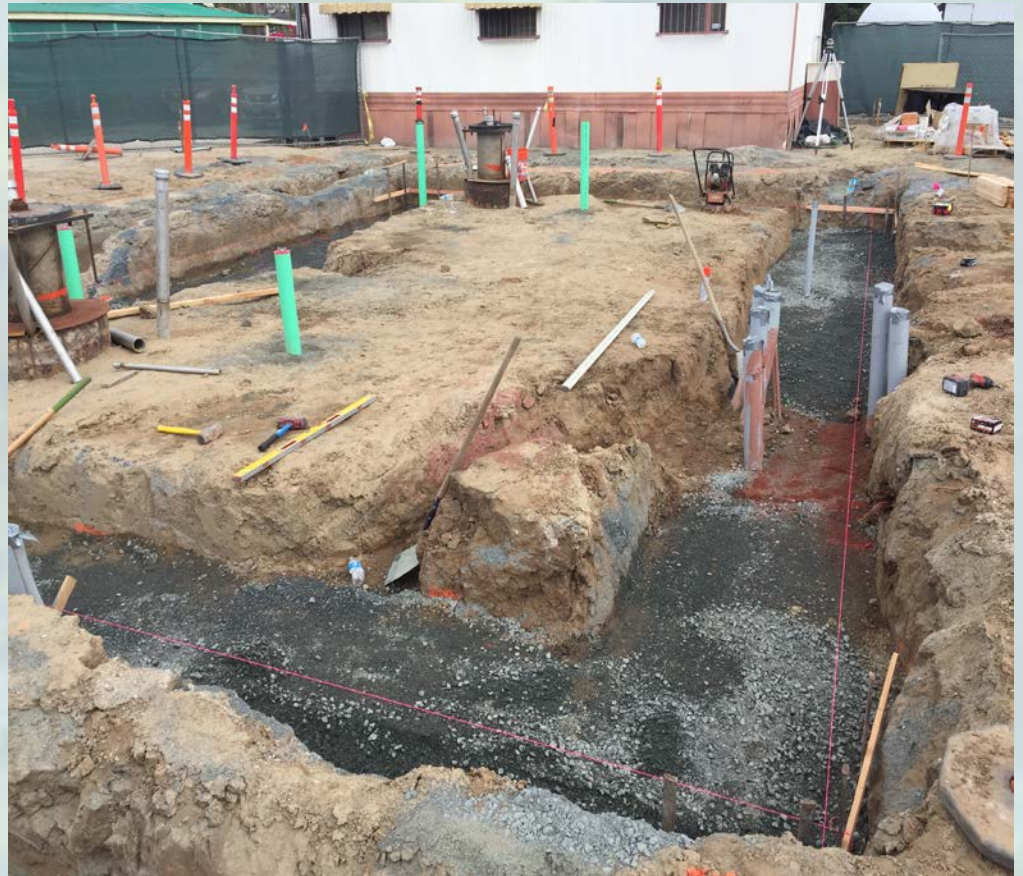
CONDUIT AND FLOOR DRAINS CONSTRUCTED
