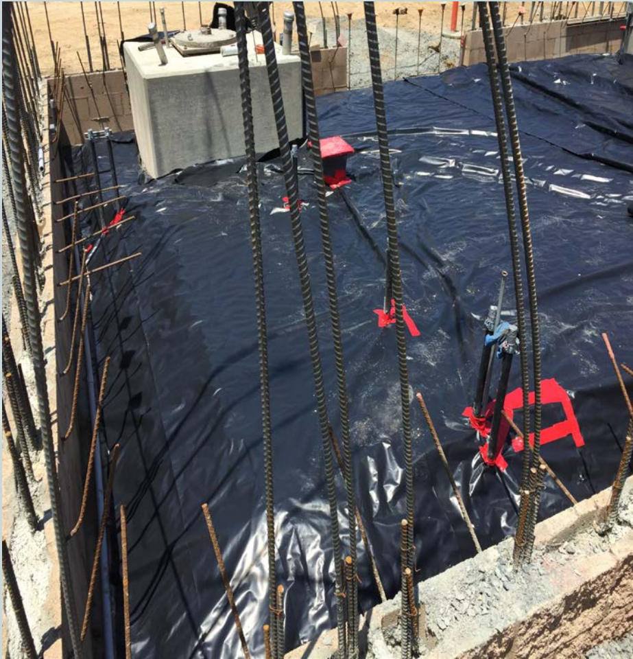
FLOOR SLAB PREPARATION
