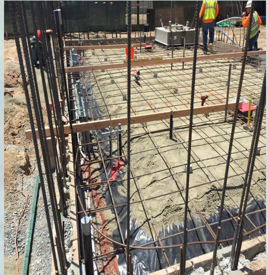
FLOOR SLAB FORMS & REINFORCING STEEL
