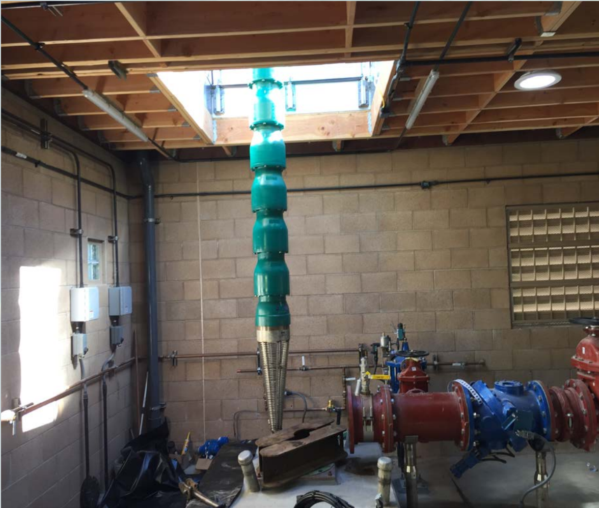
WELL 33 PUMP INSTALLATION
