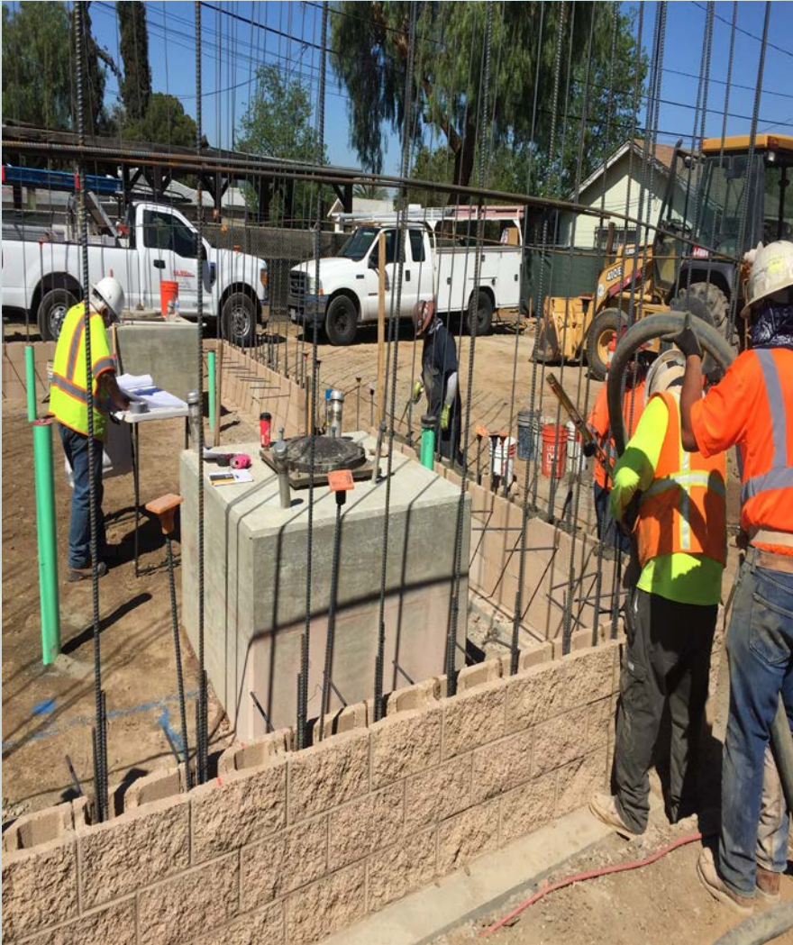
BLOCK WALL AND WELLHEADS CONSTRUCTION
