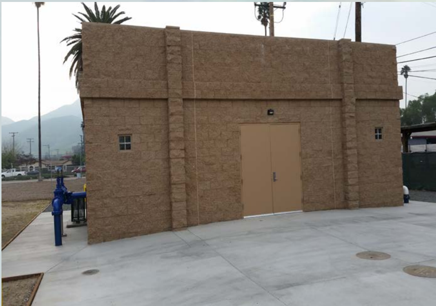
PUMP HOUSE EXTERIOR
