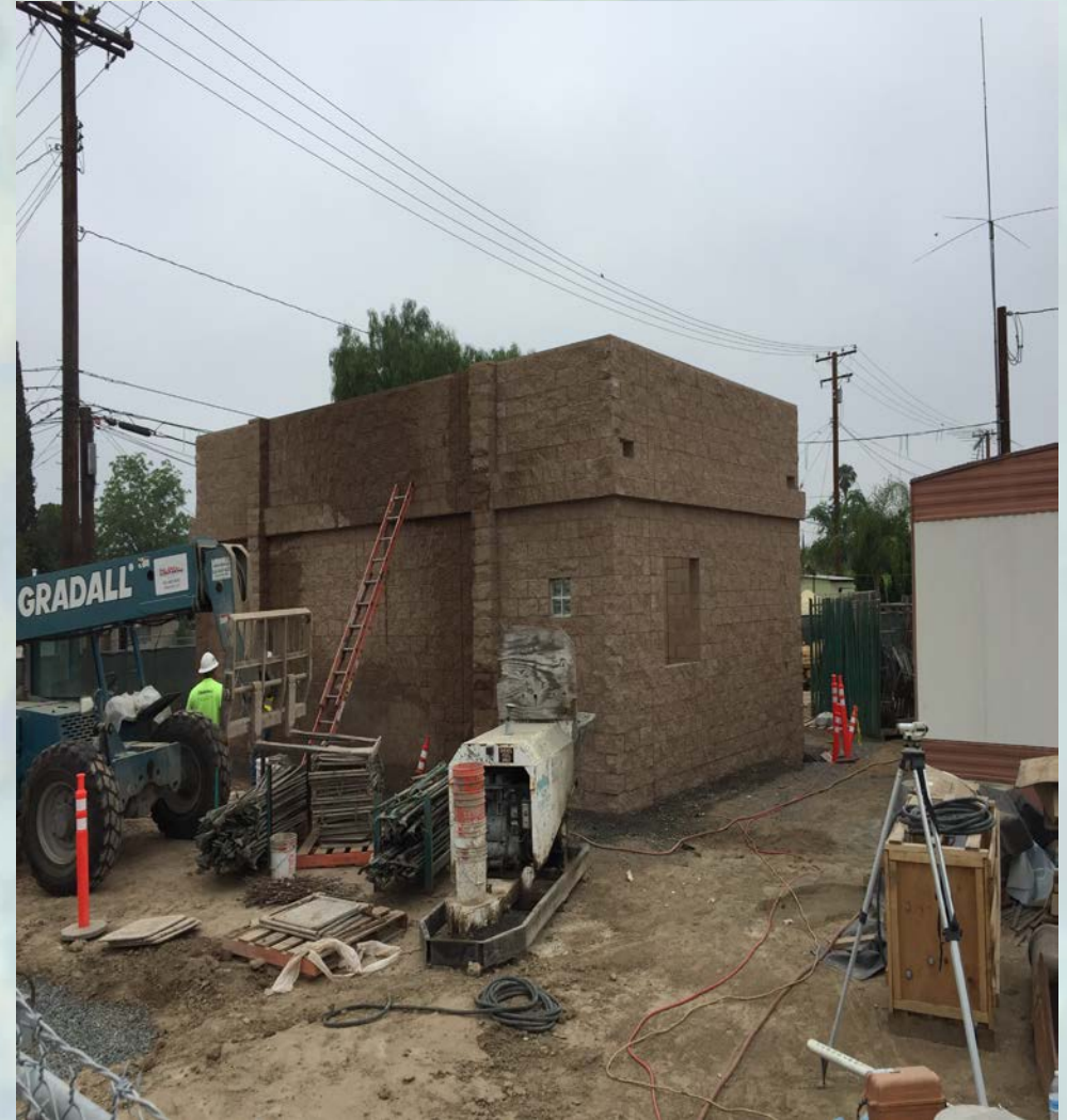
BLOCK WALL PUMP HOUSE
