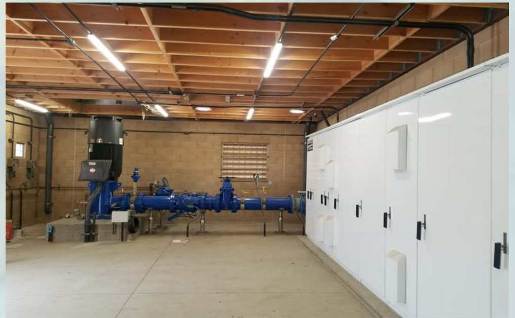
PUMP HOUSE INTERIOR
