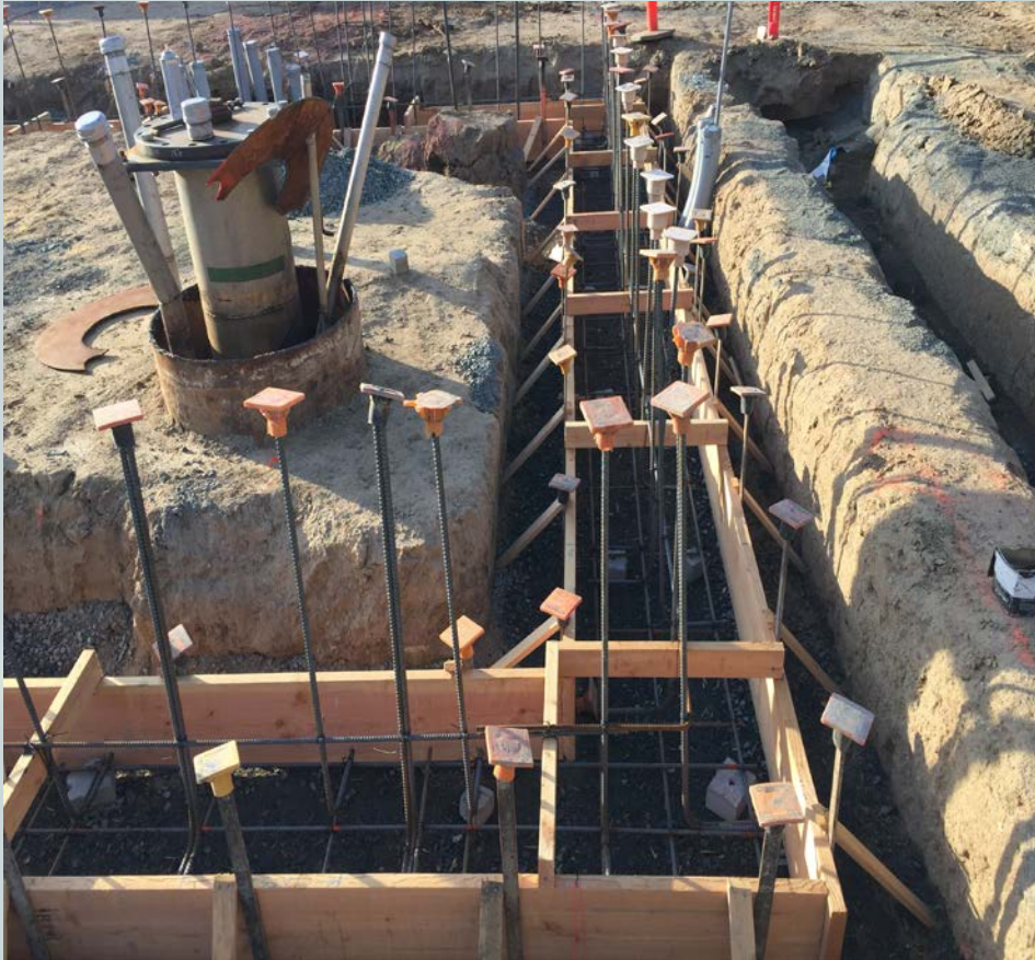
REINFORCING STEEL & FORMS FOR PUMP HOUSE FOUNDATION – WELL CASING EXPOSED
