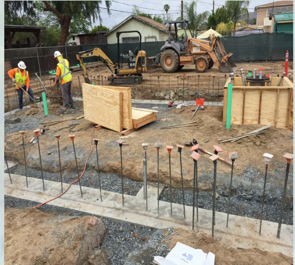
FORMING WELLHEADS FINISHED FOUNDATION W/ DOWELS FOR BLOCK WALL
