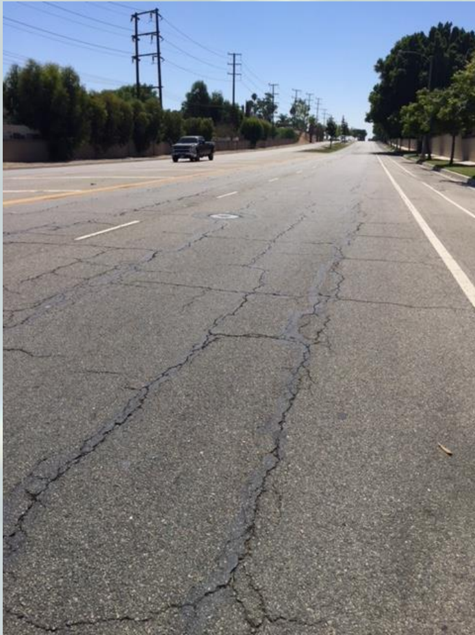
BEFORE CONSTRUCTION River Road Corona, CA
