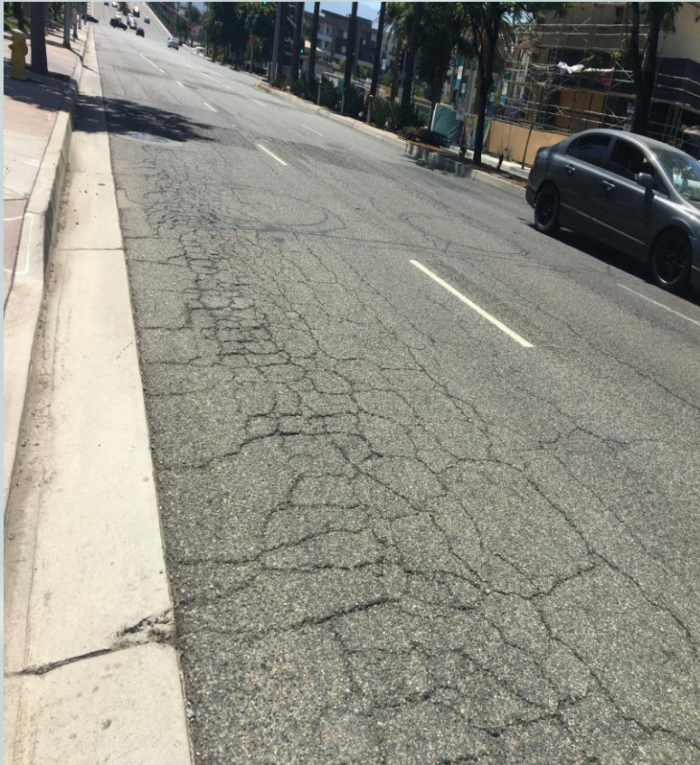
BEFORE CONSTRUCTION North Main Street Corona
