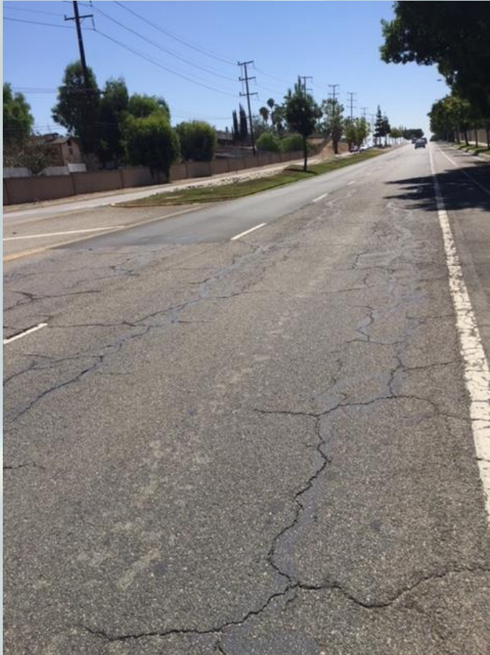
BEFORE CONSTRUCTION River Road Corona, CA
