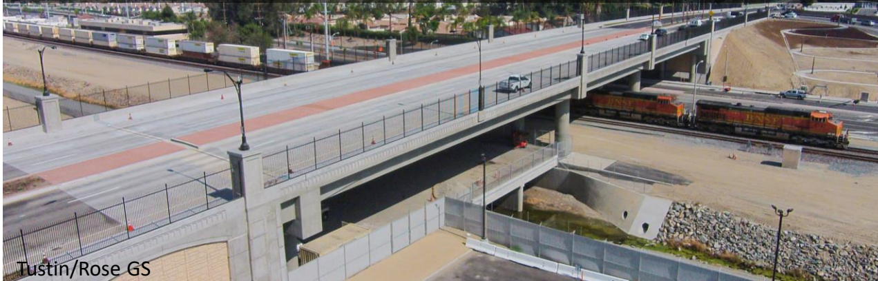
ROAD OVER RAIL (Overpass)
