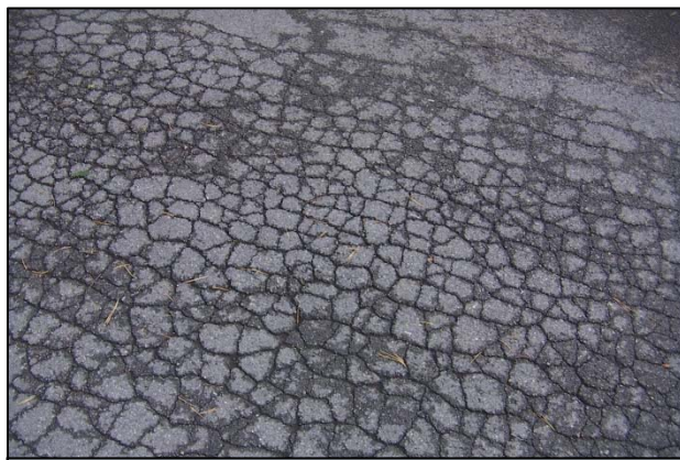
Alligator Cracking
