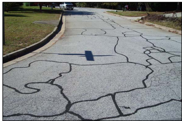
Block Cracking
