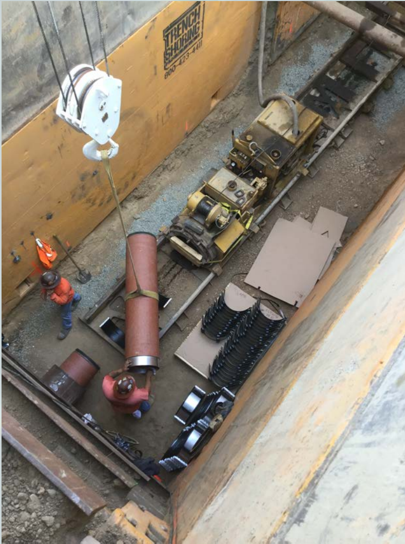
SEWER INSTALLATION IN STEEL CASING OLD TEMESCAL ROAD
