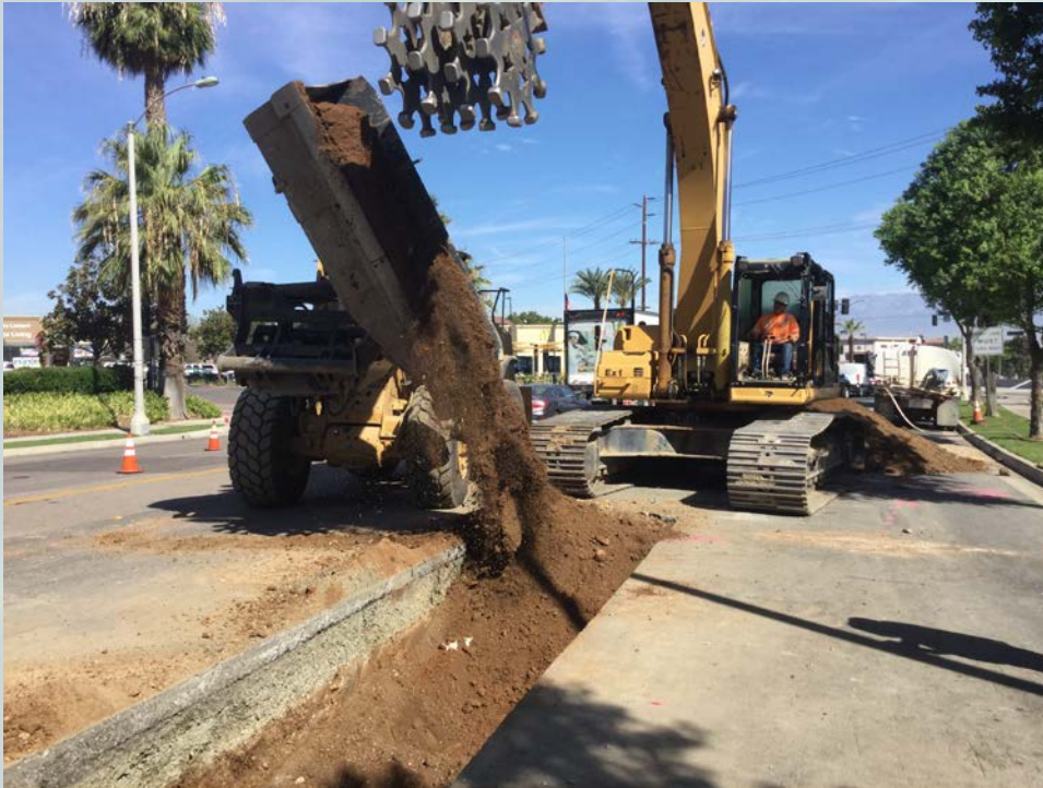
TRENCH BACKFILL
