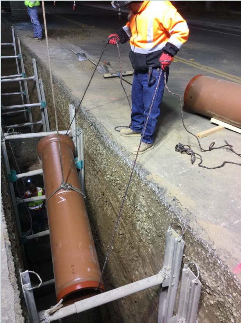
PORTIONS OF THE PROJECT WERE CONSTRUCTED AT NIGHT
