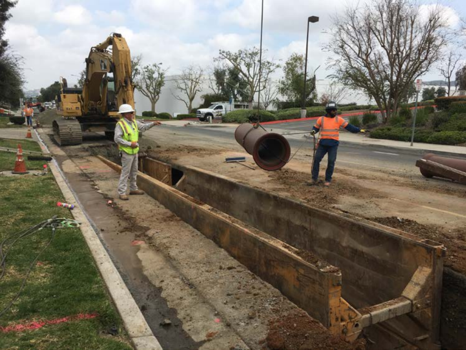
SEWER CONSTRUCTION NEAR HOME DEPOT
