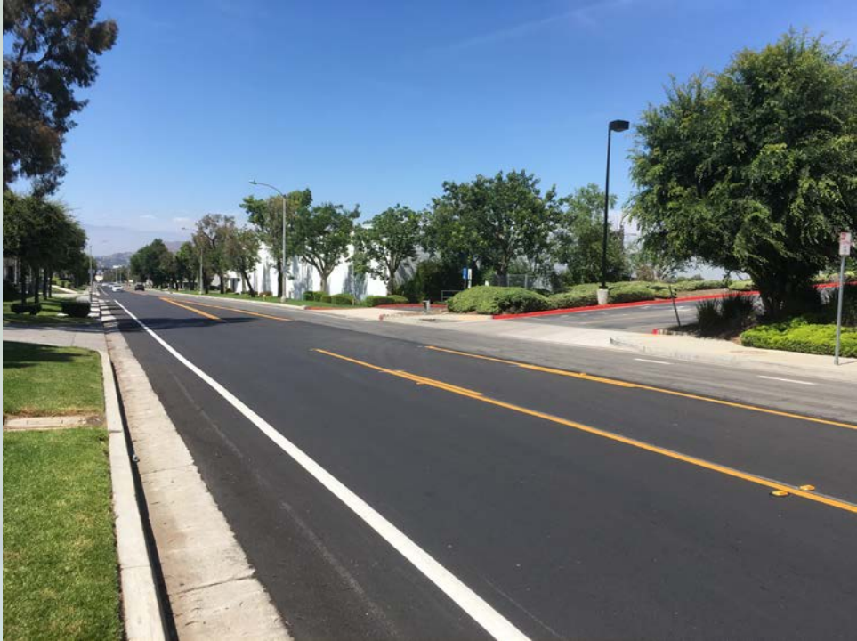
FINISH PAVEMENT NEAR HOME DEPOT
