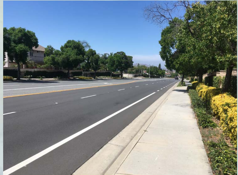
CALIFORNIA AVENUE AT CHEROKEE ROAD FINISH PAVEMENT
