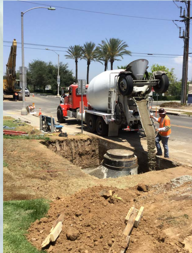
MANHOLE CONSTRUCTION AT OLD TEMESCAL ROAD
