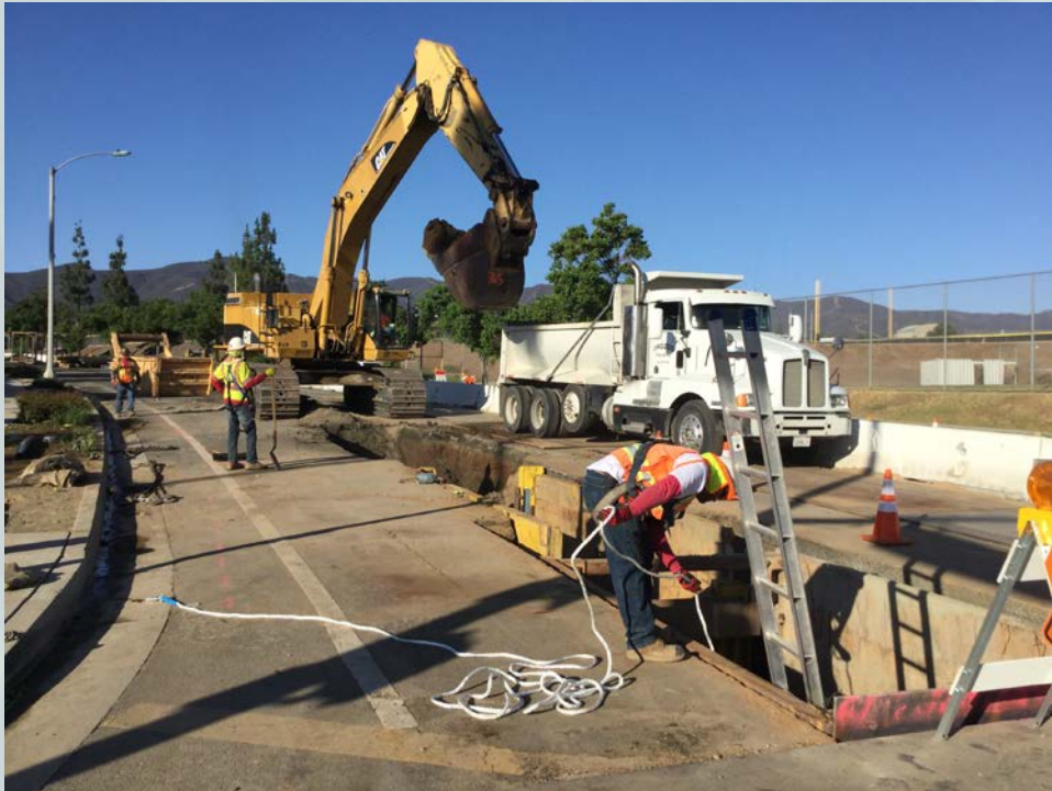
TRENCHING AND PIPE INSTALLATION NEAR CHASE DRIVE
