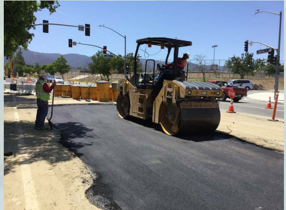
PAVING NEAR CHASE DRIVE
