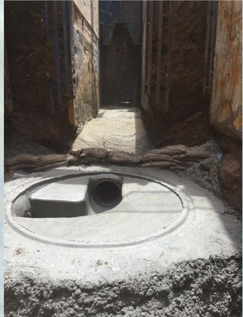
MANHOLE BASE FORMED AND READY FOR MANHOLE CONSTRUCTION
