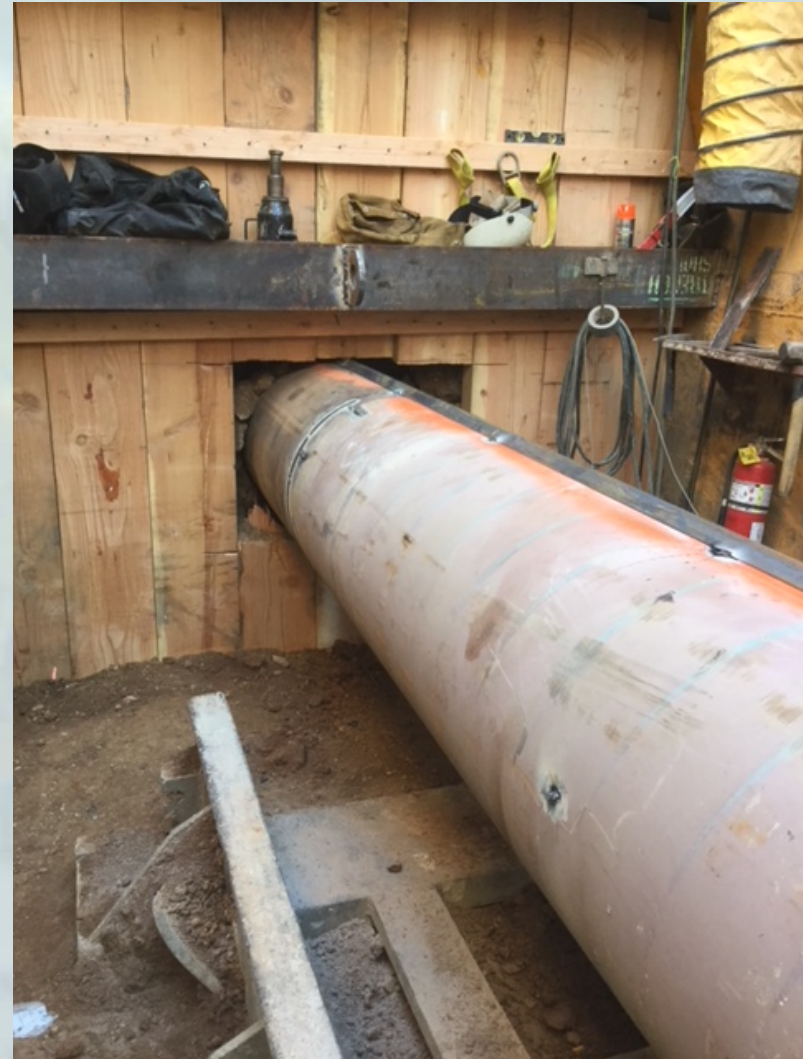
STEEL CASING INSTALLATION OLD TEMESCAL ROAD
