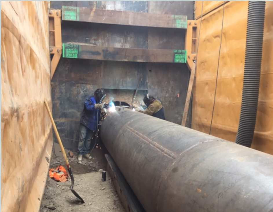
WELDING 42-INCH STEEL CASING SECTIONS
