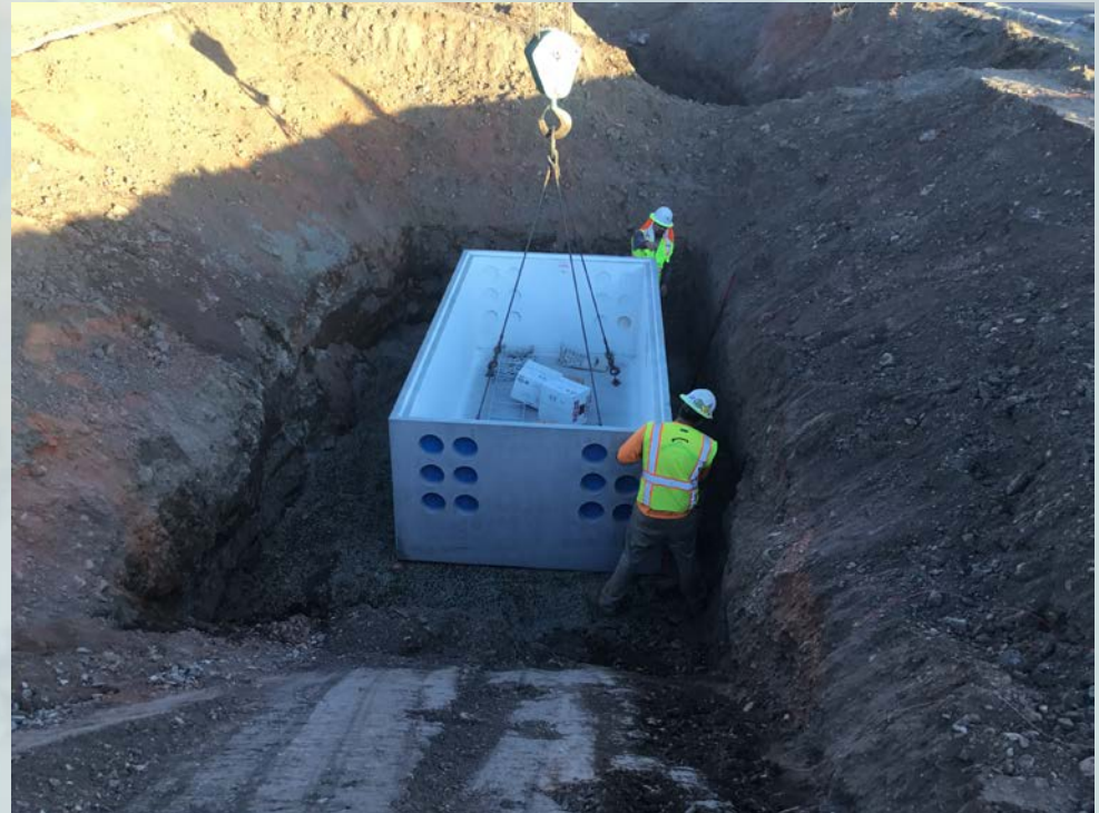
ELECTRIC VAULT INSTALLATION
