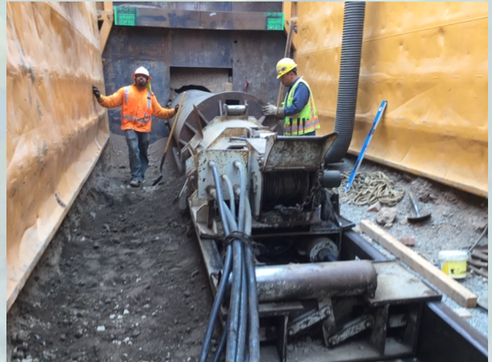
BORE & JACK STEEL CASING BENEATH BEDFORD WASH
