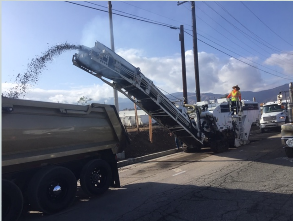
MILL AND OVERLAY PAVEMENT REPAIR
