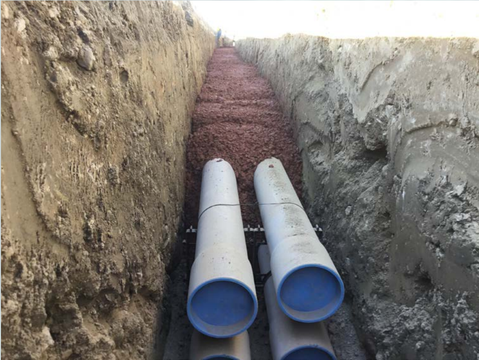
INSTALLATION OF ELECTRIC CONDUIT WITH ENCASEMENT
