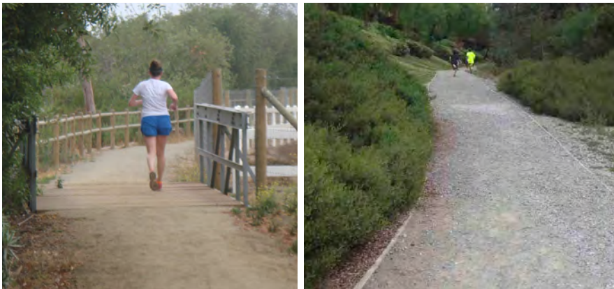
A Type 4 Trail surface needs to be compacted to be considered usable by bikes or wheelchairs..
