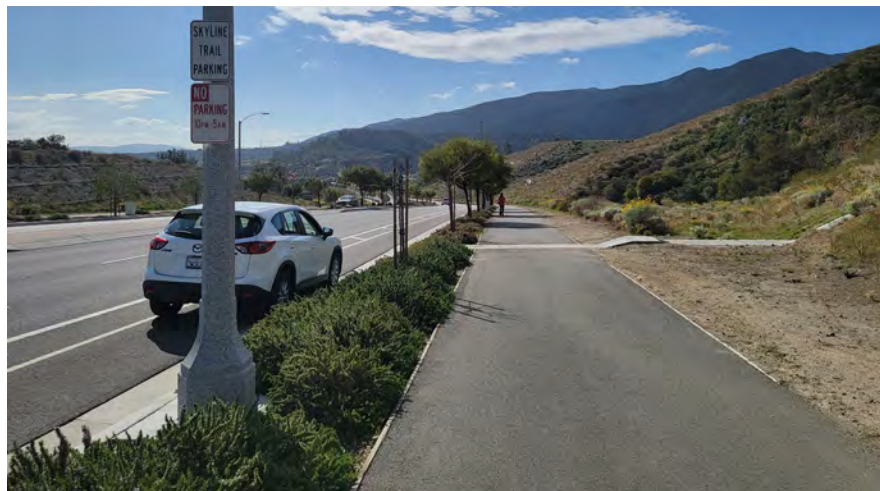
Paved multi-use path with a landscaped 5' buffer from the edge of the road
