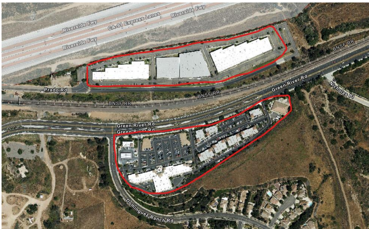
4225 -4375 Prado and 4180-4350 Green River: Properties in High Fire Severity Zones in Corona.
