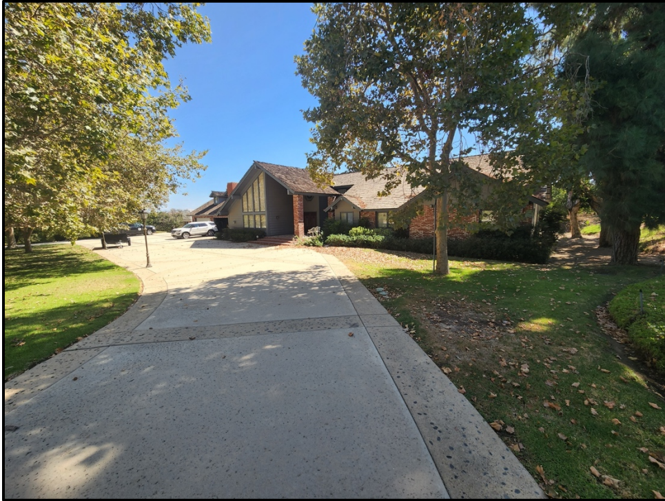
Plate 4.2–2: Overview of the residence on the property, facing northeast.
