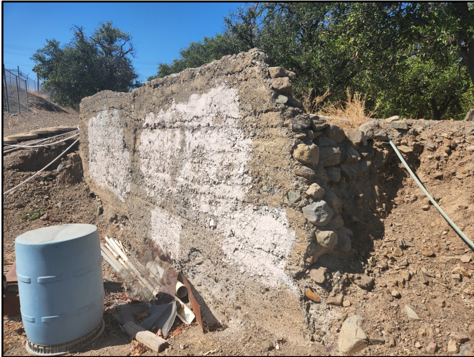
Plate 4.2–4: Overview of the rock and mortar retaining wall, facing south.
