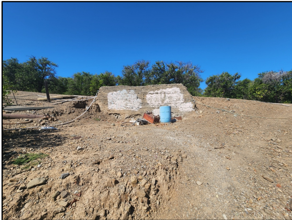
Plate 4.2–3: Overview of rock and mortar retaining wall, facing west.
