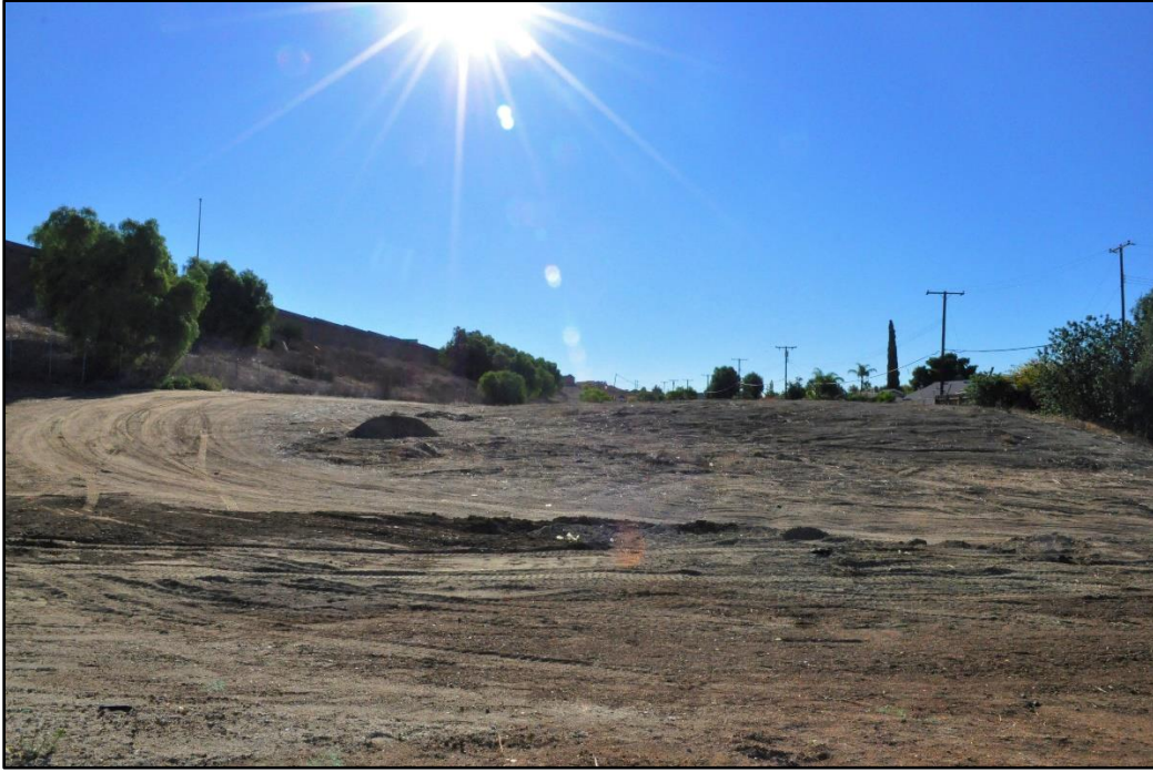
Figure 1. View of the site from the northwest boundary of the Project area near Corona Avenue
