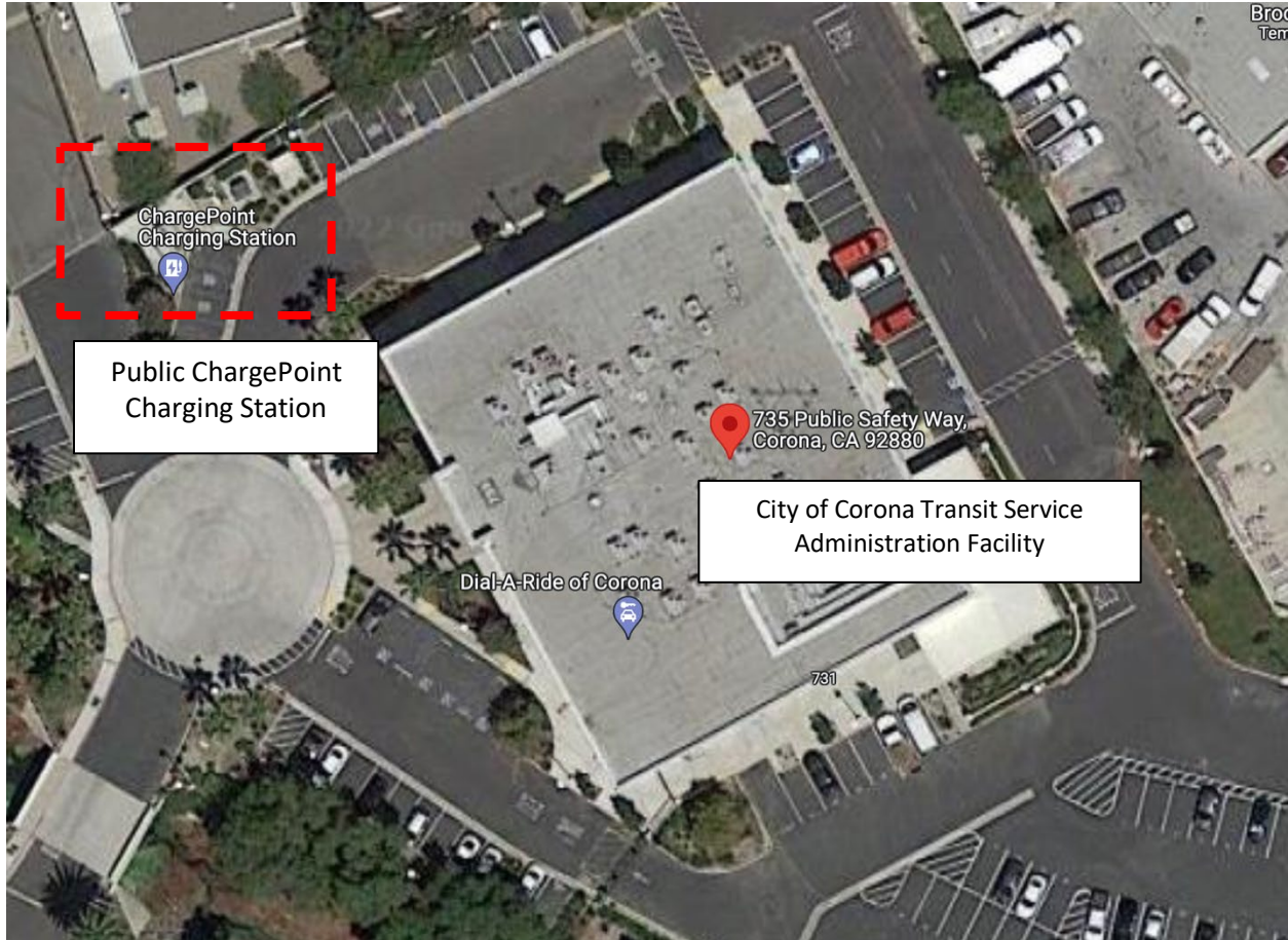
Figure 3 – CCTS Administrative and Maintenance Facility
