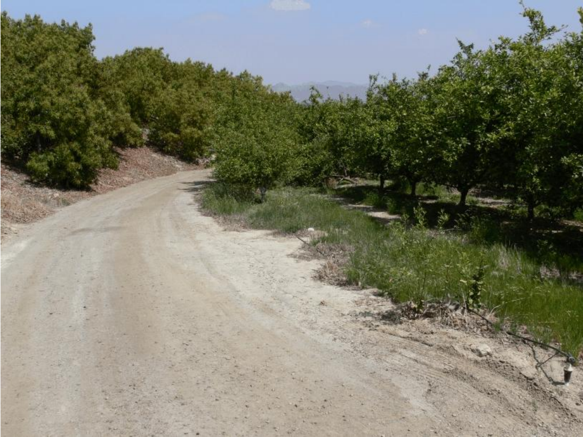
Drain D (photo 21): The head of Drain D begins to the right of the lemon tree next to the road near the center of the photo.
