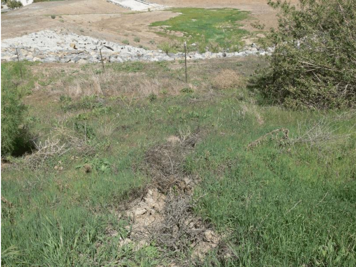
Drain B (photo 12): End of Drain B showing an incised drainage in the foreground. The chain-link fence in the background is the property border with a drainage basin beyond that.
