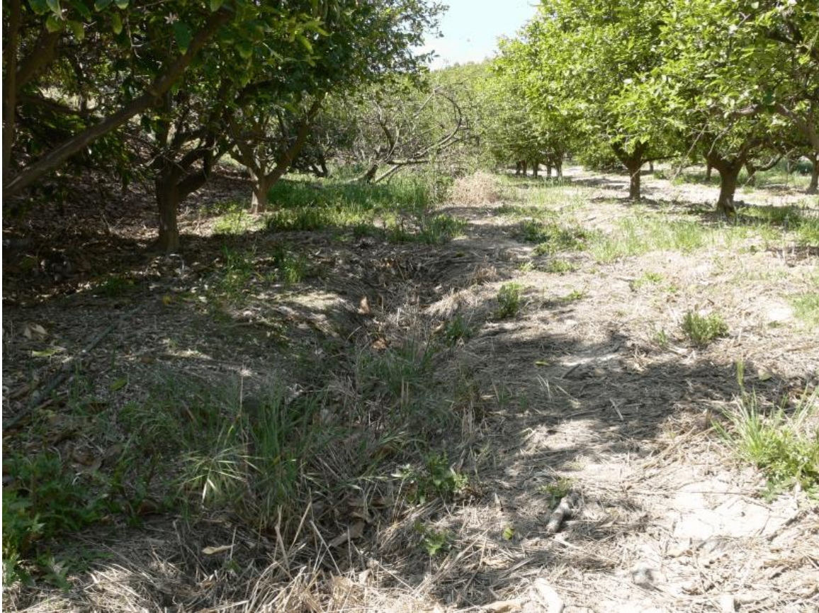
Drain D (photo 22): This photo shows typical conditions along one of the drainage branches that make up Drain D as it passes between rows of lemon trees.
