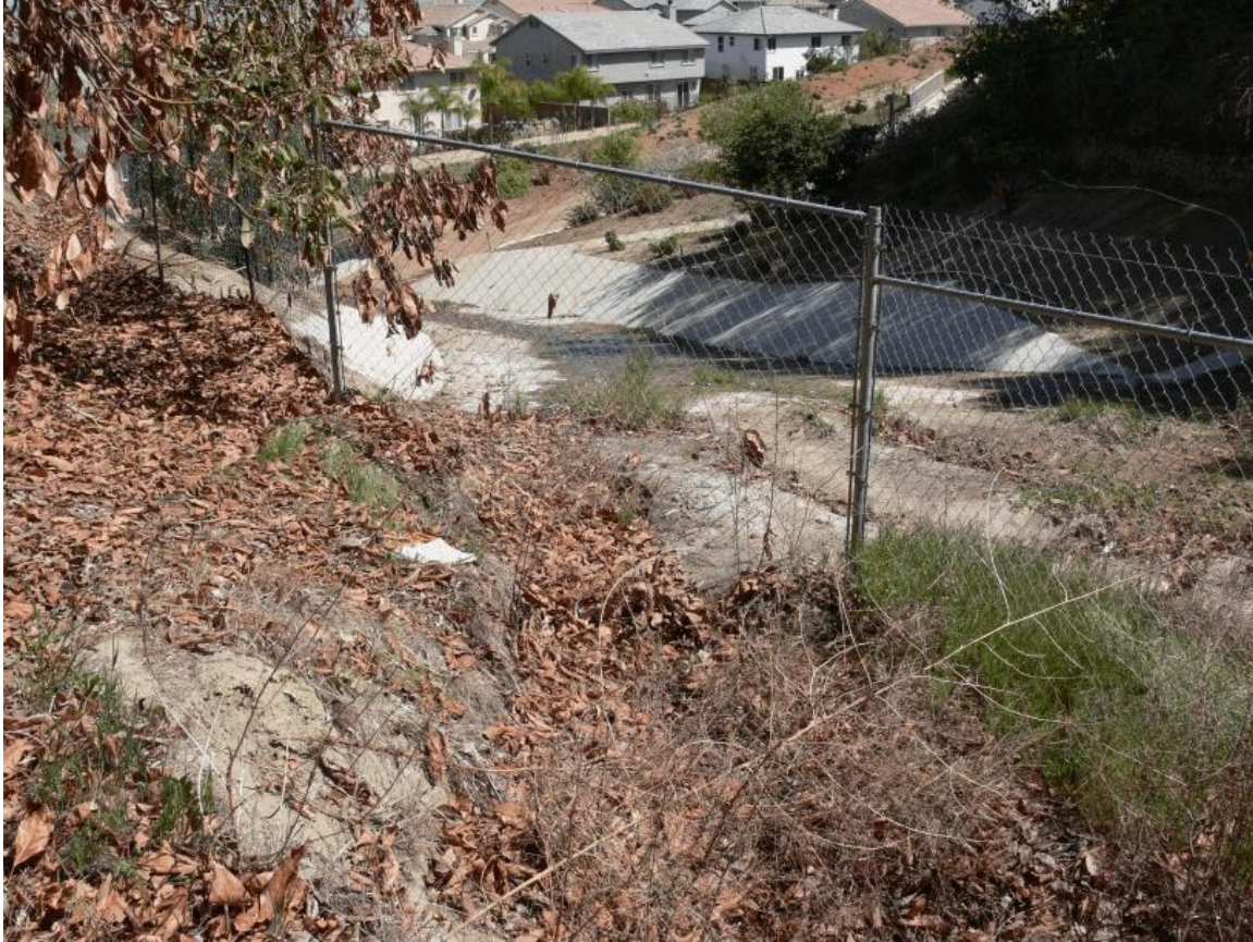
Drain A (photo 5): Location where Drain A leaves the site and enters cement lined channel to basin along north edge of subject property.
