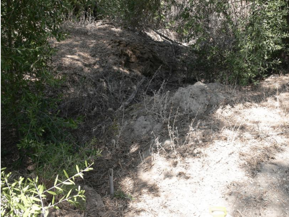
Drain F (photo 30): The drainage continues off site on the west side of the road (lower right corner of the photo).
