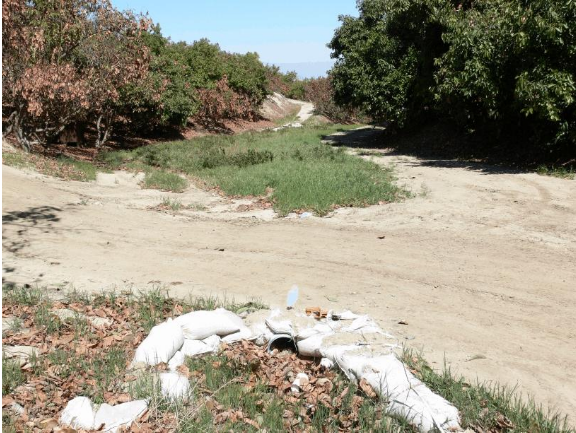
Drain B (photo 11): Looking north from just south of location of previous photo. Drainage passes through pipe under road into this grassy area before leaving the property.
