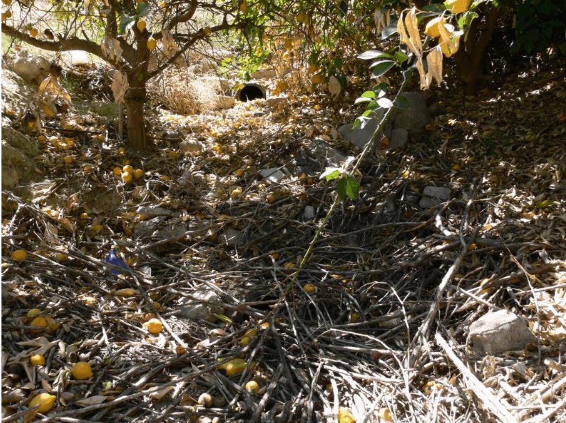
Drain C (photo 14): The pipe opening onto the property can be seen as the dark oval shape in the background of this photo taken looking to the south. The drainage passes through the center of a stand of lemon trees in a leaf and branch strewn path. The drainage passes through the lower left corner of the photo.
