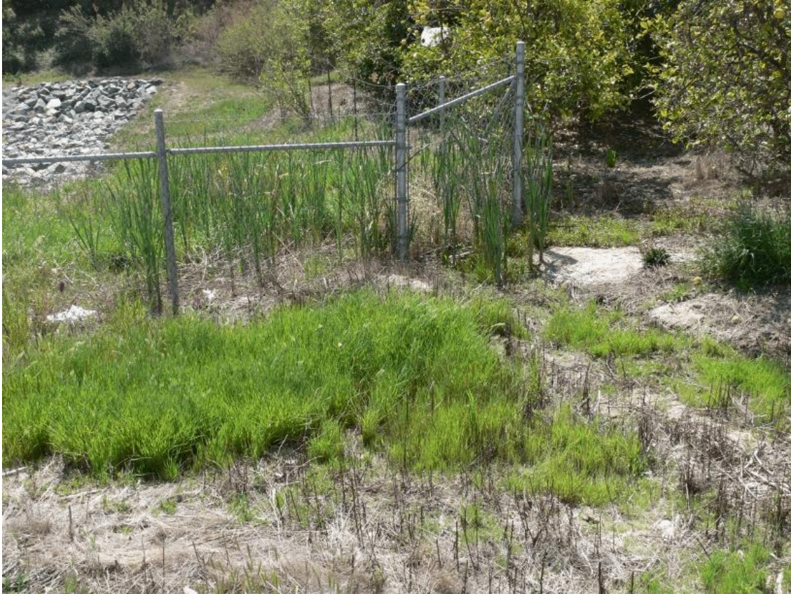
Drain D (photo 24): Drainage D leaves the site at this fence separating the subject property from the drainage basin beyond. Runoff from orchard irrigation has formed a wet area here and just beyond the fence.
