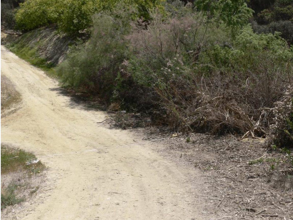
Drain C (photo 13): Drain C enters the property through a pipe under this road from the patch of mule fat on the right side of the photo. The white measuring tape on the road marks the approximate location of the pipe.
