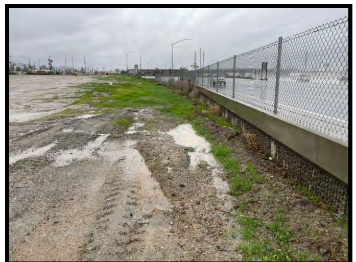
Photo #6: View looking west along north property line.
