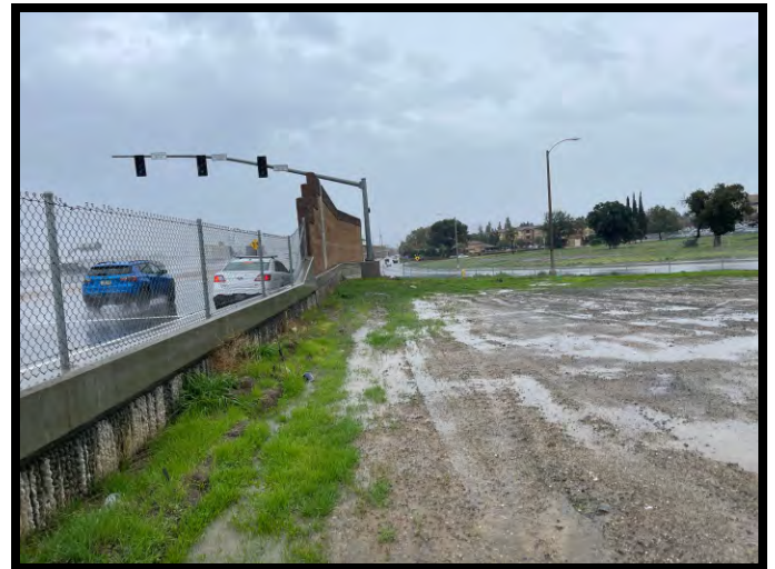
Photo #4: View looking east along freeway wall.
