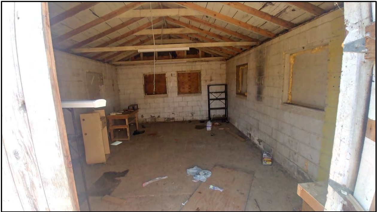
Plate 4.2–9: Interior view of the cinderblock garage at Site Temp-1.
