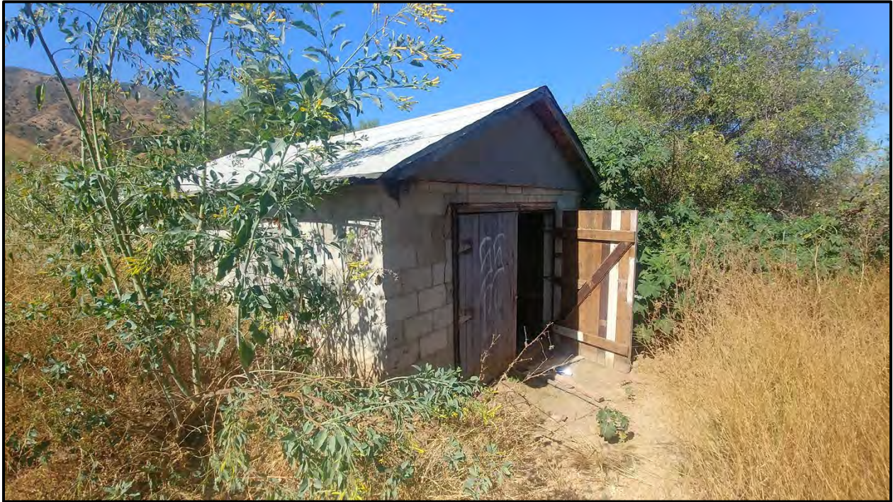
Plate 4.2–8: Overview of the north (primary) and east façades of the cinderblock garage at Site Temp-1, facing southwest.
