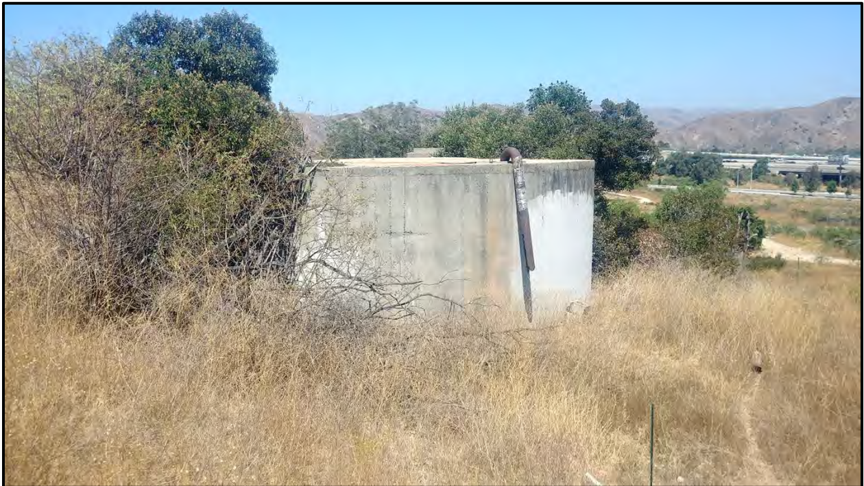
Plate 4.2–7: Close-up view of the board-formed concrete water tank at Site Temp-1, facing northwest.
