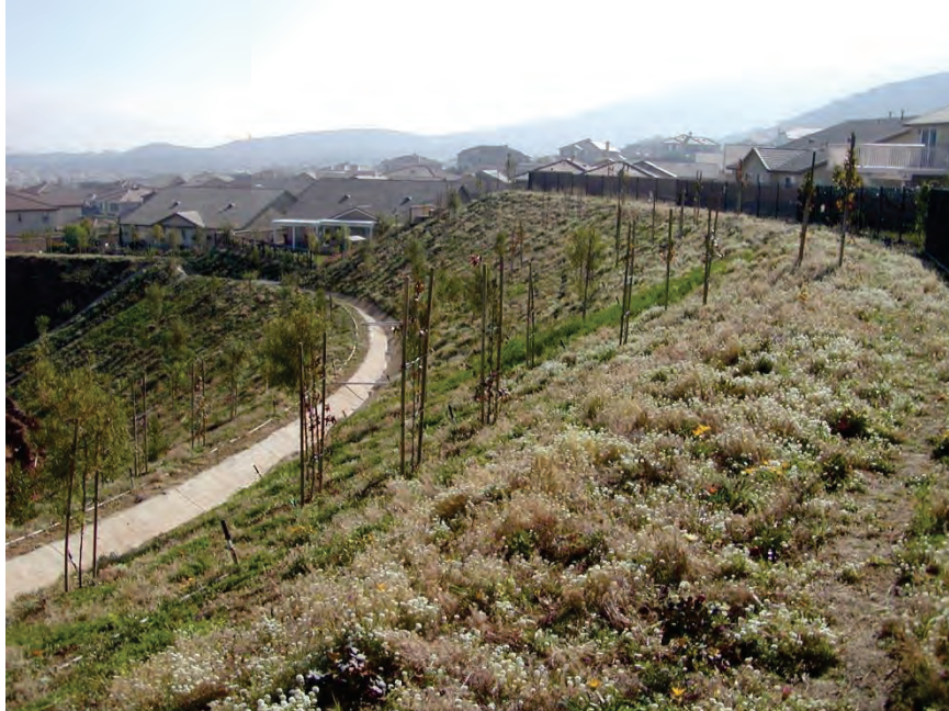
Photo #6 - An Example of a Manufactured Slope That is Irrigated or Temporarily Irrigated Until Plant Establishment.
