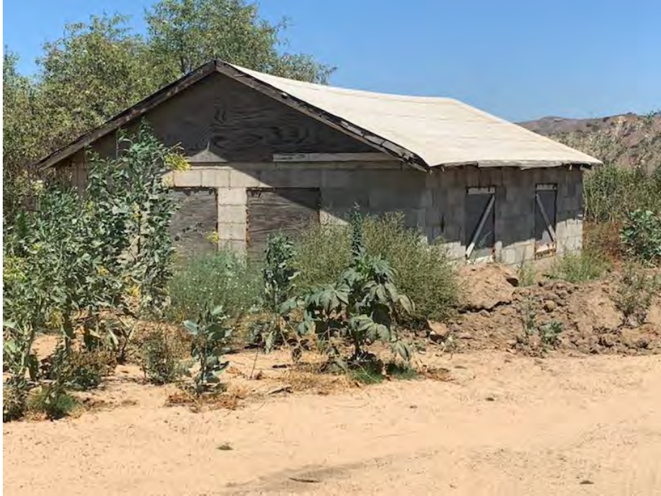
7. View north from northeast portion of site.
