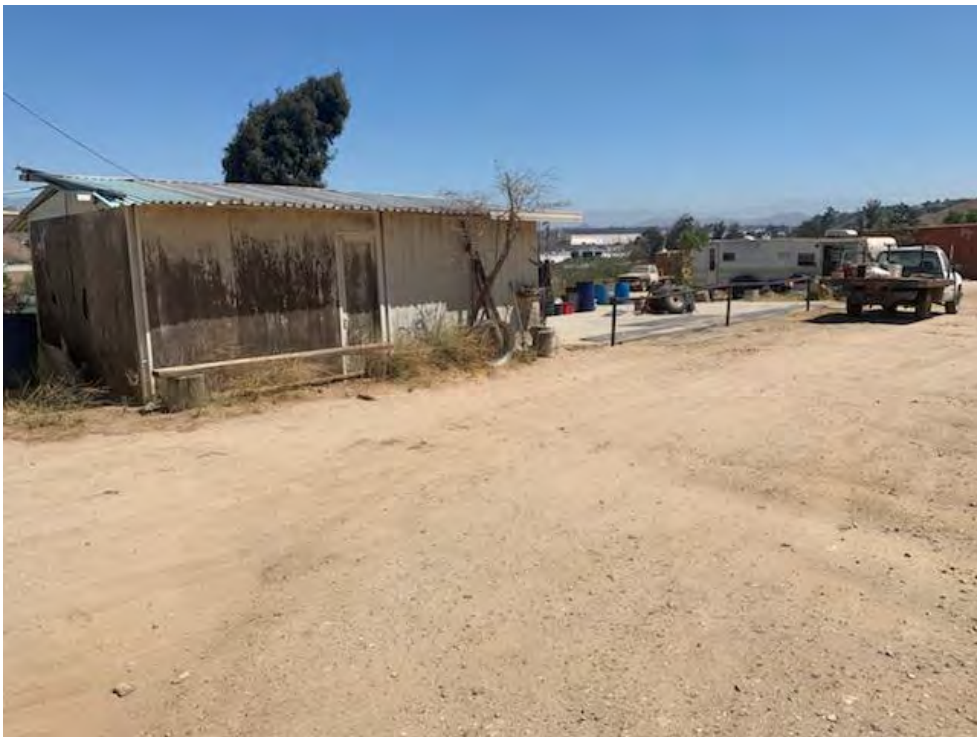
10. View northwest from northeast portion of the site.
