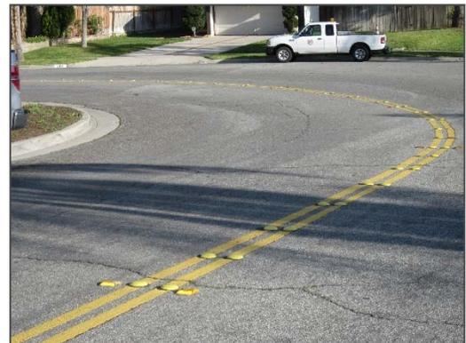
and approved by the City Traffic Engineer, raised pavement markers (RPM)'s, also known as a "bot dots", will be added to the striping to assist motorist in staying in their lane.
