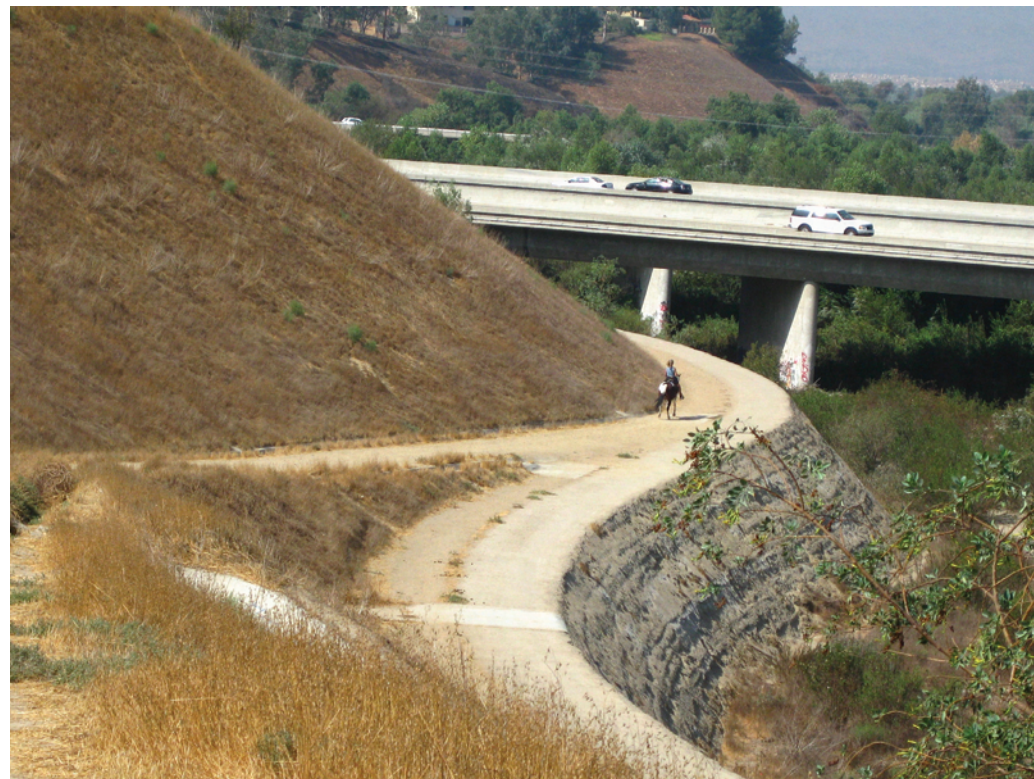
The recommended soft surface trail in Norco will be located on the USACE bench out of the flood plain.
