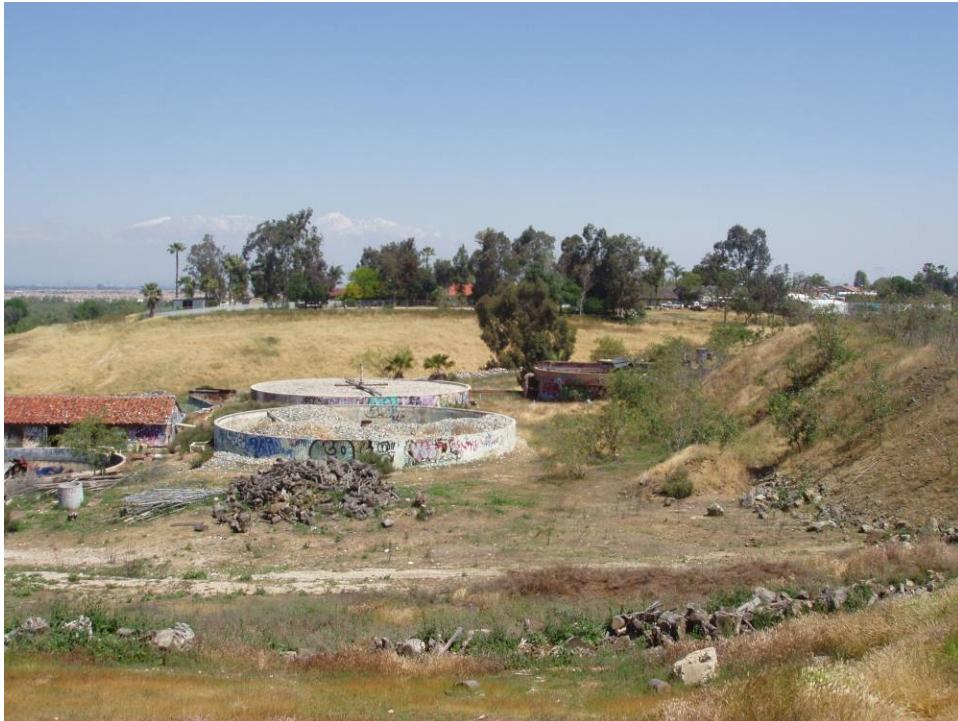
Photograph 6: View of an unrecorded historic water waste treatment plant north of Norco Drive in Reach IX. Most of the soils in this area are artificial due to build up of soil during developmental construction.
