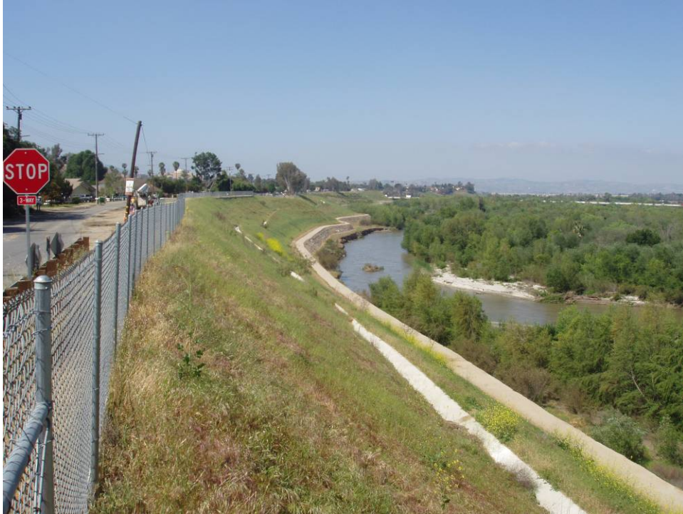
Photograph 3: Reach XI downstream view with River Road to the left. The trail shall be placed on the embankment in this photograph.
